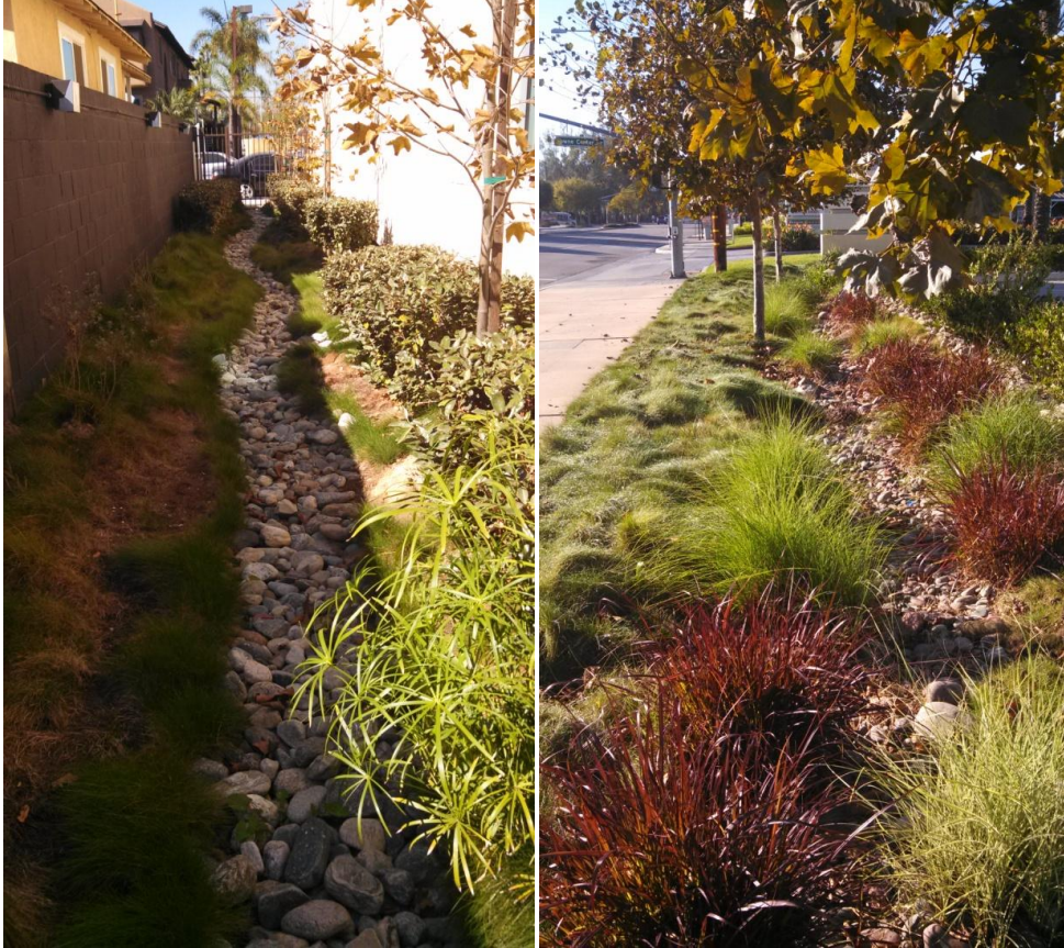
Figure 2: Vegetated Swale (Seal Beach, CA).
